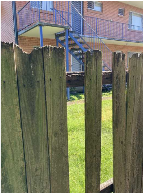
Wood rot in timber fence
