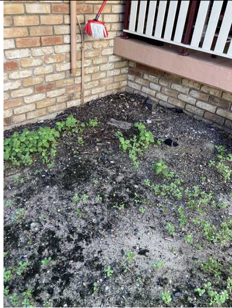
Garden beds against building walls
