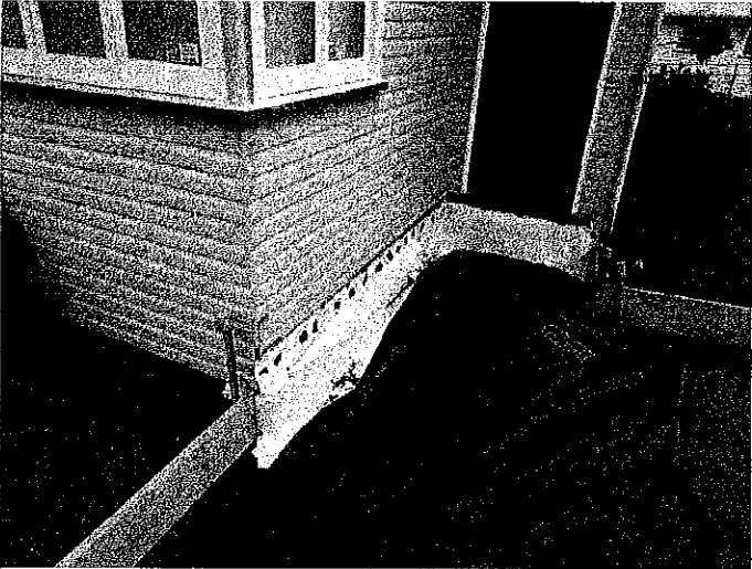
Homeguard install to 31 Herbert St, Camp Hill November 2013
