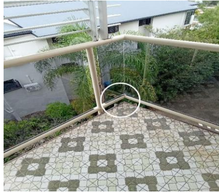
Partial detachment of rubber seal.
