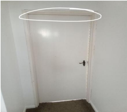
Door rubbing on head.
