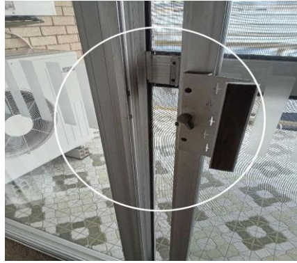
Lock not latching closed against frame.
