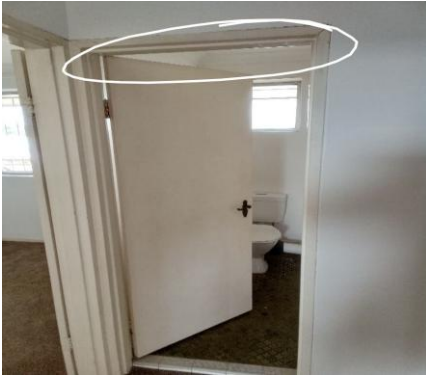
Door rubbing on top of jamb.
