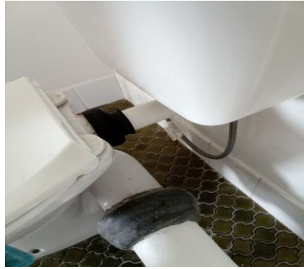
Rubber flush pipe seal brittle.
